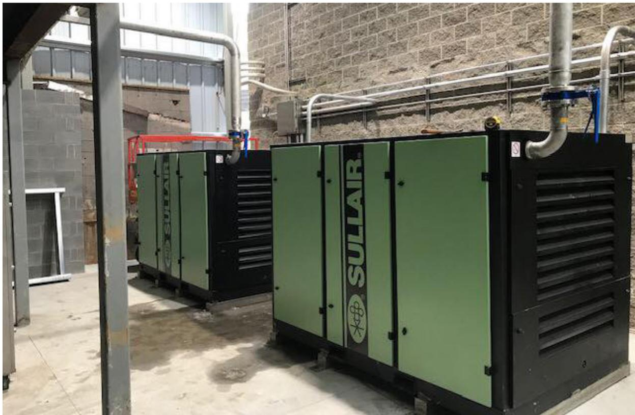
When choosing an industrial air compressor, customers are often faced with a decision to select a compressor with Spiral Valve Technology or Variable Speed Drive. There are considerations for each – with an important one being the climate and environment in which the compressor is used.
