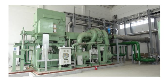
This entry discusses how the modern multi-stage integrally geared centrifugal compressor has a wide range of pressures, flow, and turndown and can be used as both a baseload and for trimming compressor applications.
