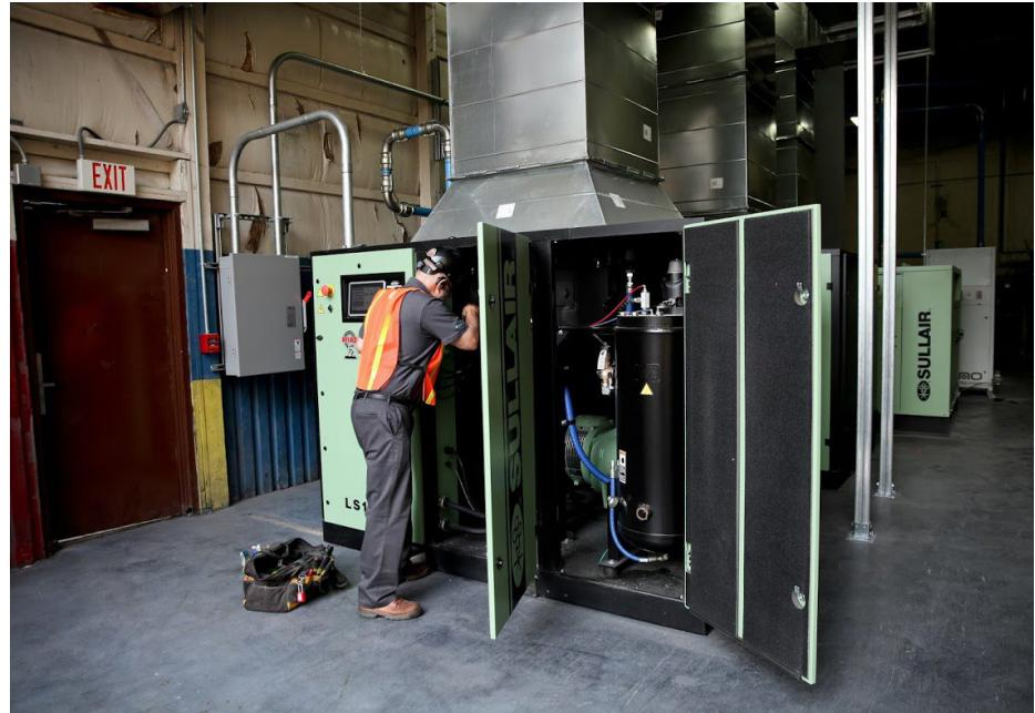
Atlas Machine & Supply Sullair service technician works on an LS Series compressor
