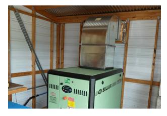
Additionally, you do not want to install an industrial air compressor in an area with a high amount of particulate. That can clog a cooler and cause overheating.
